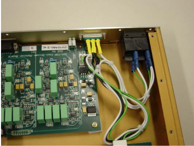
Figure 7: UIM PP Chassis Power Harness
