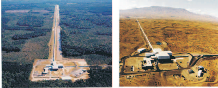
Figure 1. The LIGO sites in Livingston, Louisiana (left) and Hanford, Washington (right). The arms extend 4 km from the corner station and contain vacuum pipes so the entire optical path is in vacuum.
