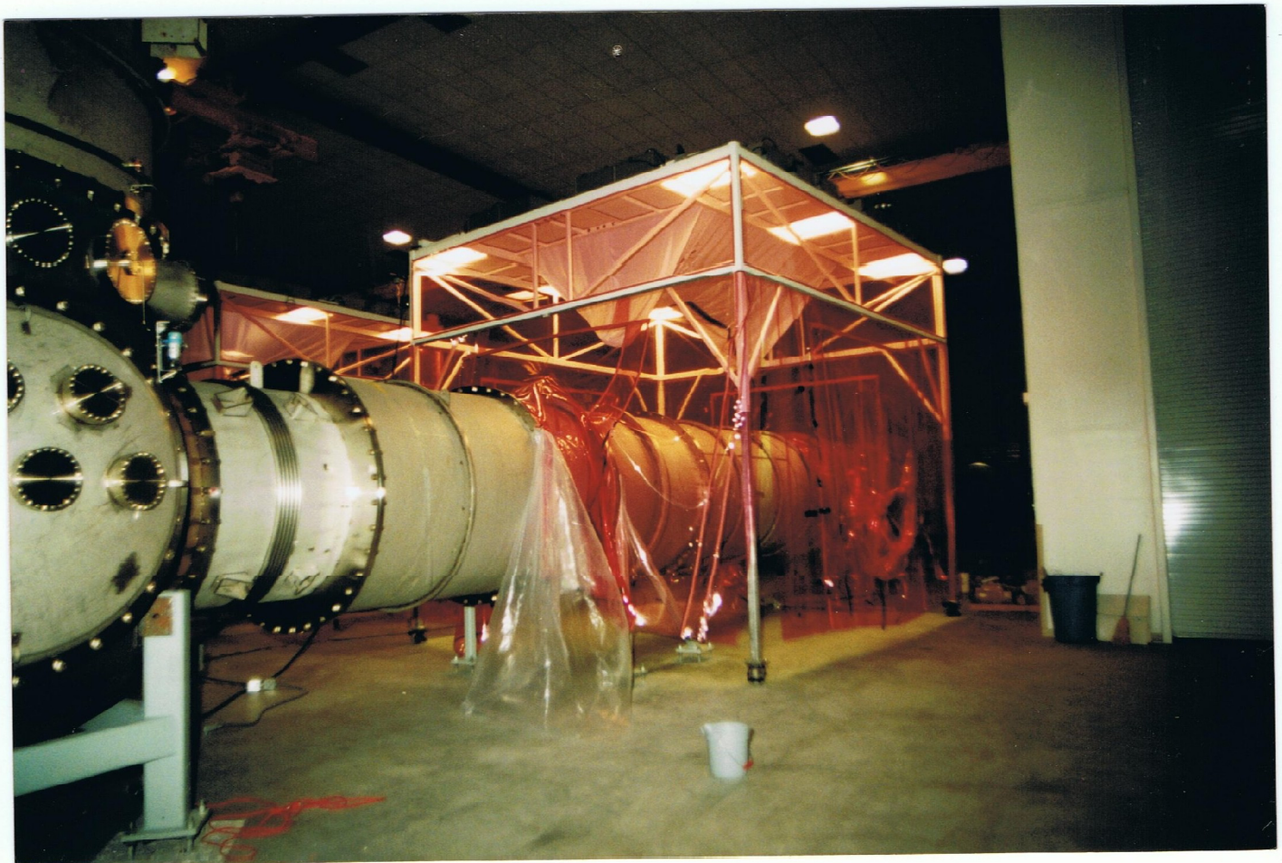
PORTABLE CLEANROOMS USED FOR INSTALLATION
