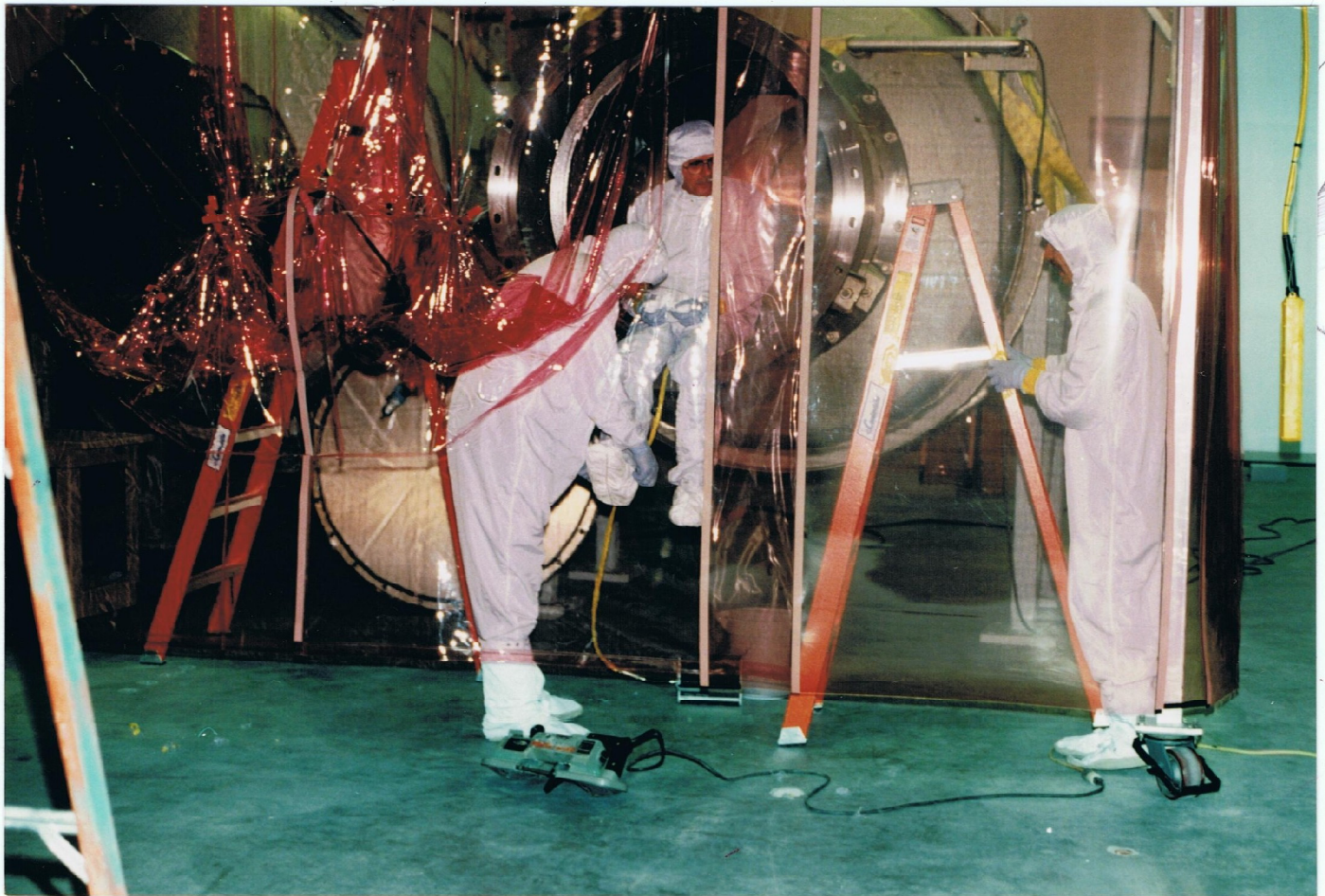
PORTABLE CLEANROOMS USED FOR INSTALLATION
