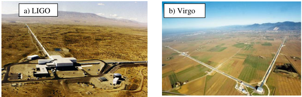
FIGURE 2. Bird's eye view a) of the LIGO detector site at Hanford (courtesy of the LIGO project) and b) of the Virgo detector site at Cascina in Italy (courtesy of the Virgo project).
