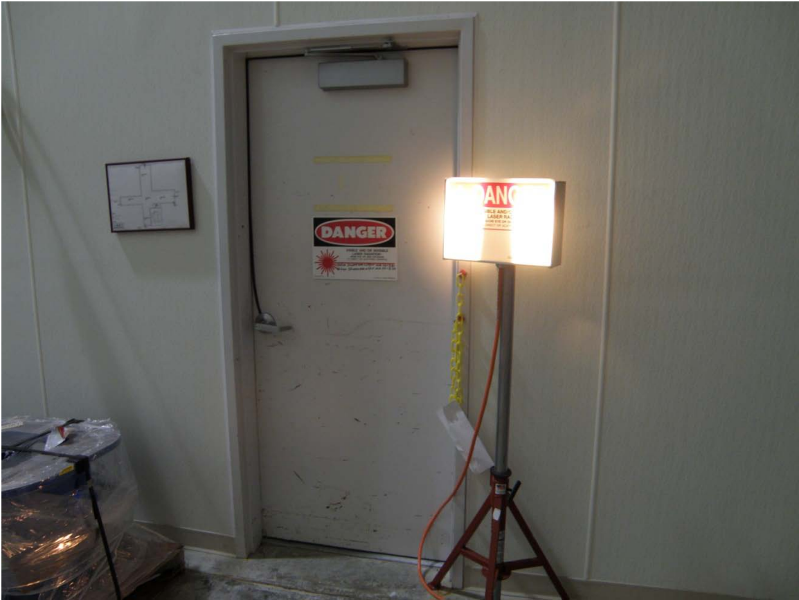
Figure 2: An example of a portable illuminated sign on the right. A posted unlit sign can be seen on the door. This photo was taken in the LVEA large airlock.
