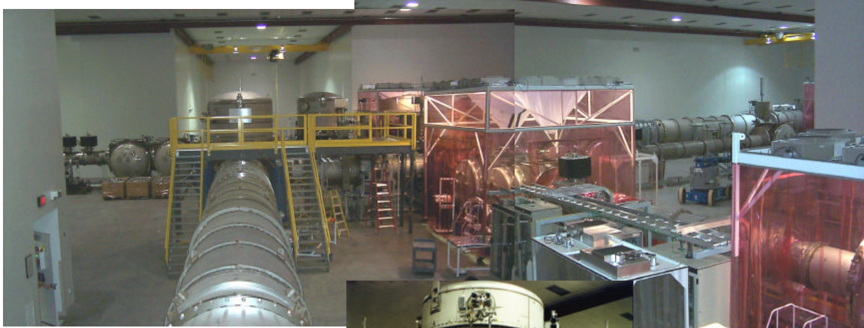
View inside Corner Station
