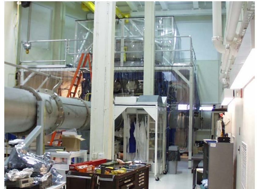
BSC chamber including cartridge clean room
