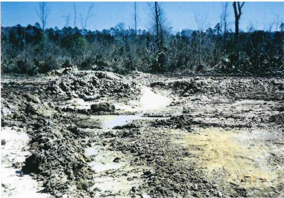
19.Southeast Arm showing a temporary drain ditch to assist in the removal of rain water from the berm area.
