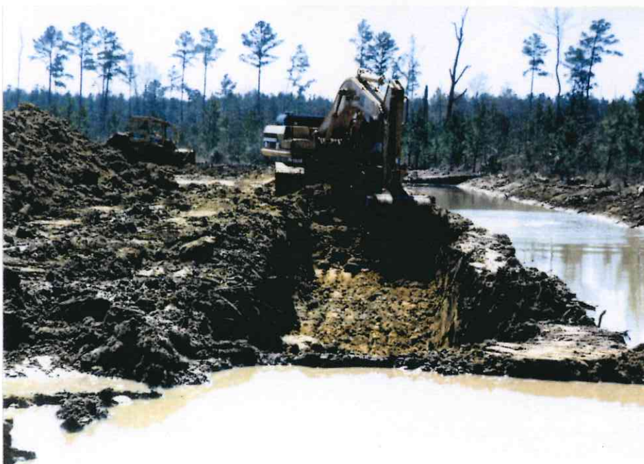
12. Southeast arm at station 131+00 excavating for berm fill.
