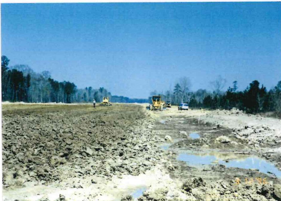
18. Southeast Arm at station 128+00 looking at the drying of berm material .
