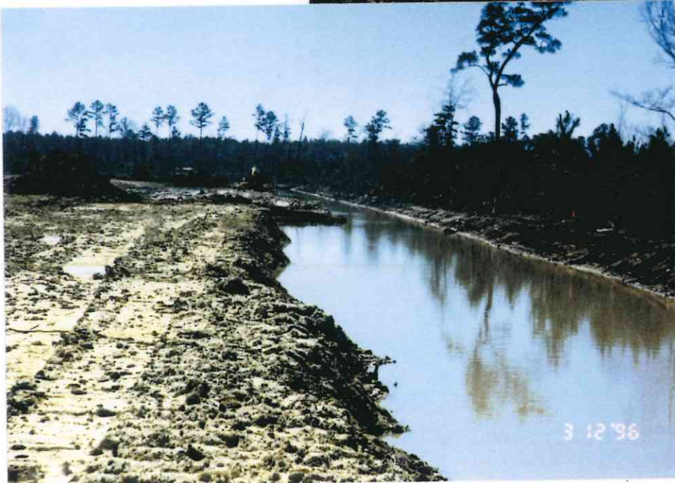
9. Southeast Arm at station 120+00 looking SE at excavating trench for berm material.
