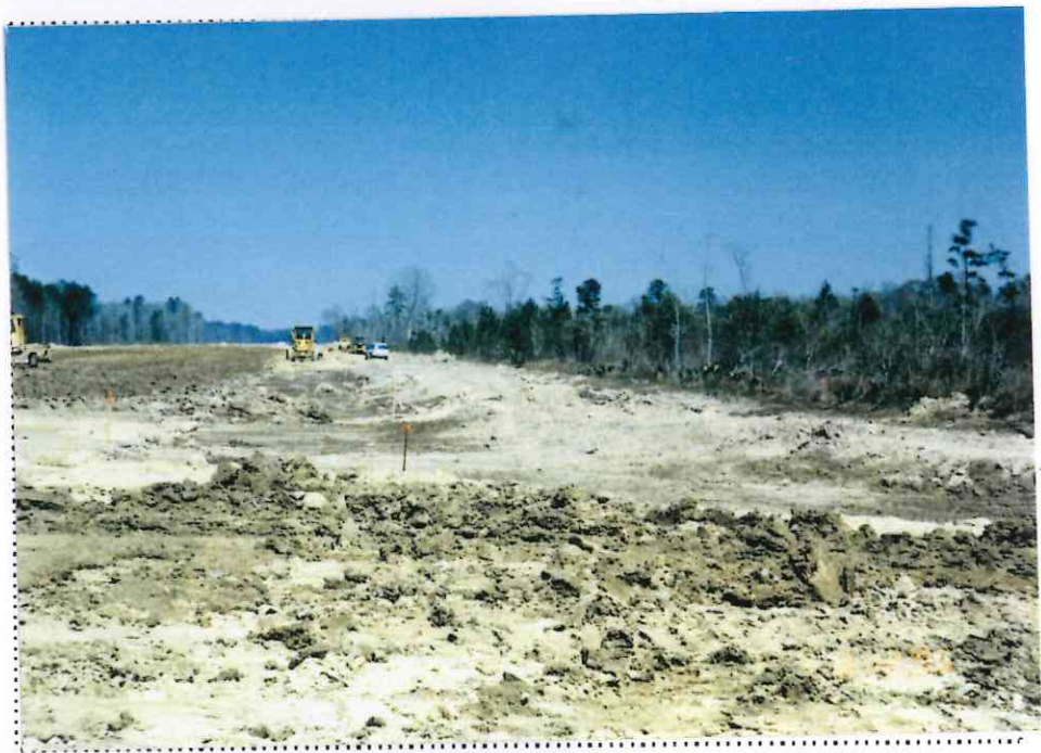
16. Southeast Arm at station 132+00 looking NW before starting disking in foreground and the disking operation on going in the background.
