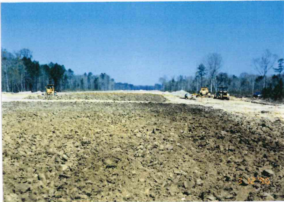
7. Southeast Arm at station 115+00 looking north at the results of diskling berm material.
