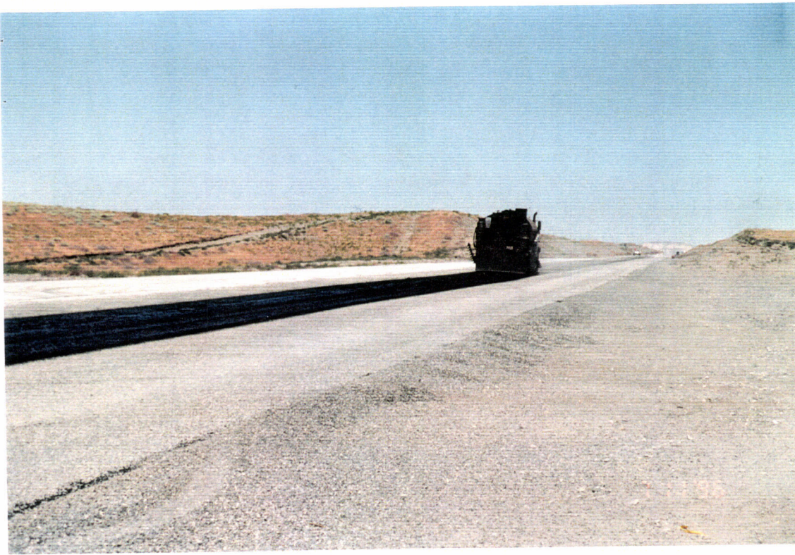
Spraying CRS-2, the second layer of multiple layer of bituminous road surfacing along the southwest arm.
