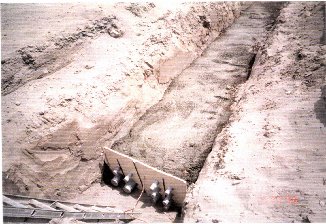
Typical duct bank at the contract interface point near the buildings.
