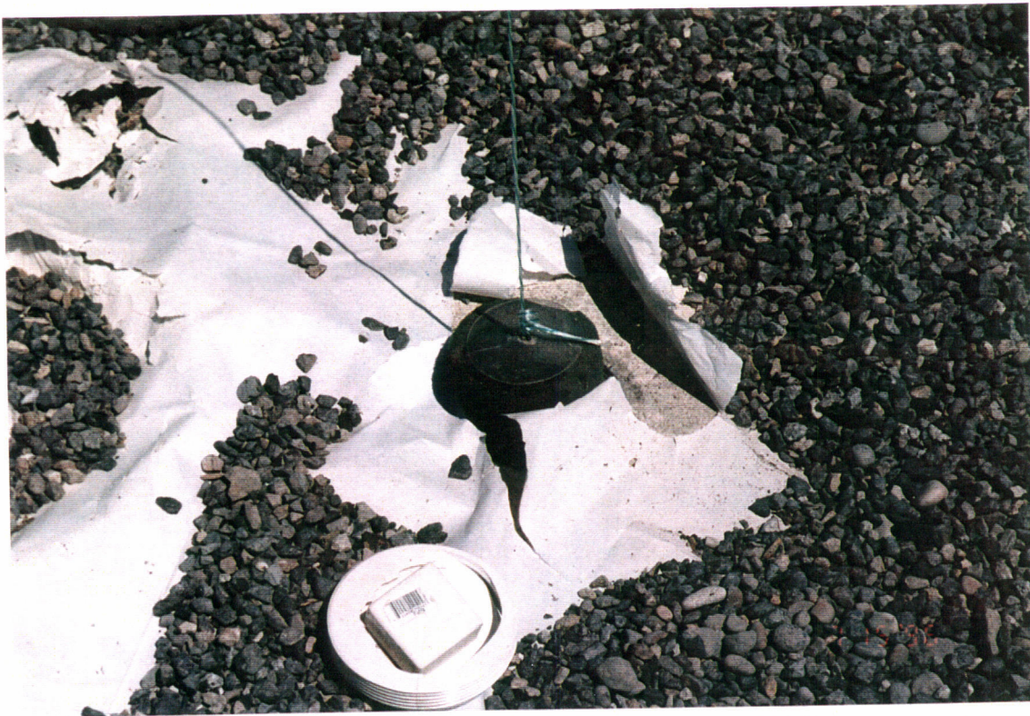
At the service entrance, verifying the integrity of the duct bank conduits and installing the pull rope for the future power cable installation.
