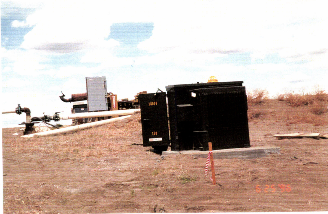
PUD provided and installed 500 kva transformer at the well No. 1.
