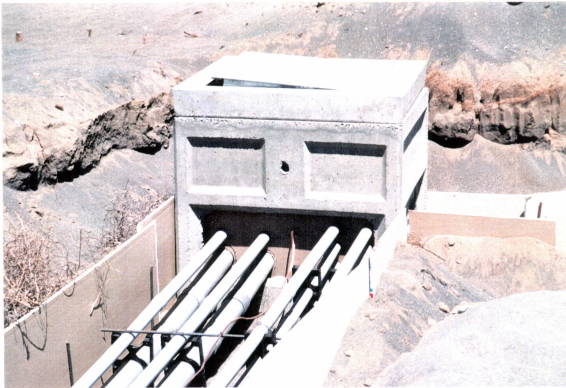
Typical electrical cable pull box and conduit penetration supply side to the southwest arm End Station.
