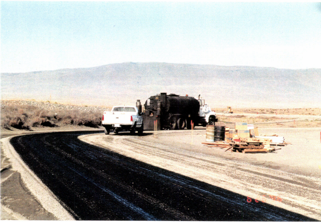
MC-250 spraying is continued along the temporary access road
