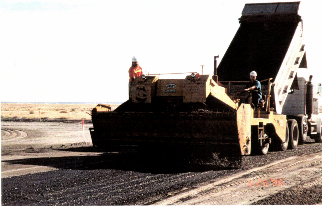
Close up view of the gravel spreading equipment.
