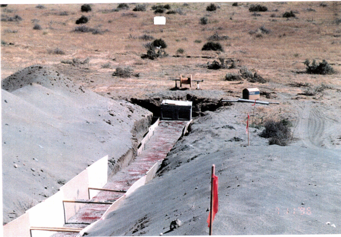
Another view of the duct bank from the southwest End Station to the electrical pull box.
