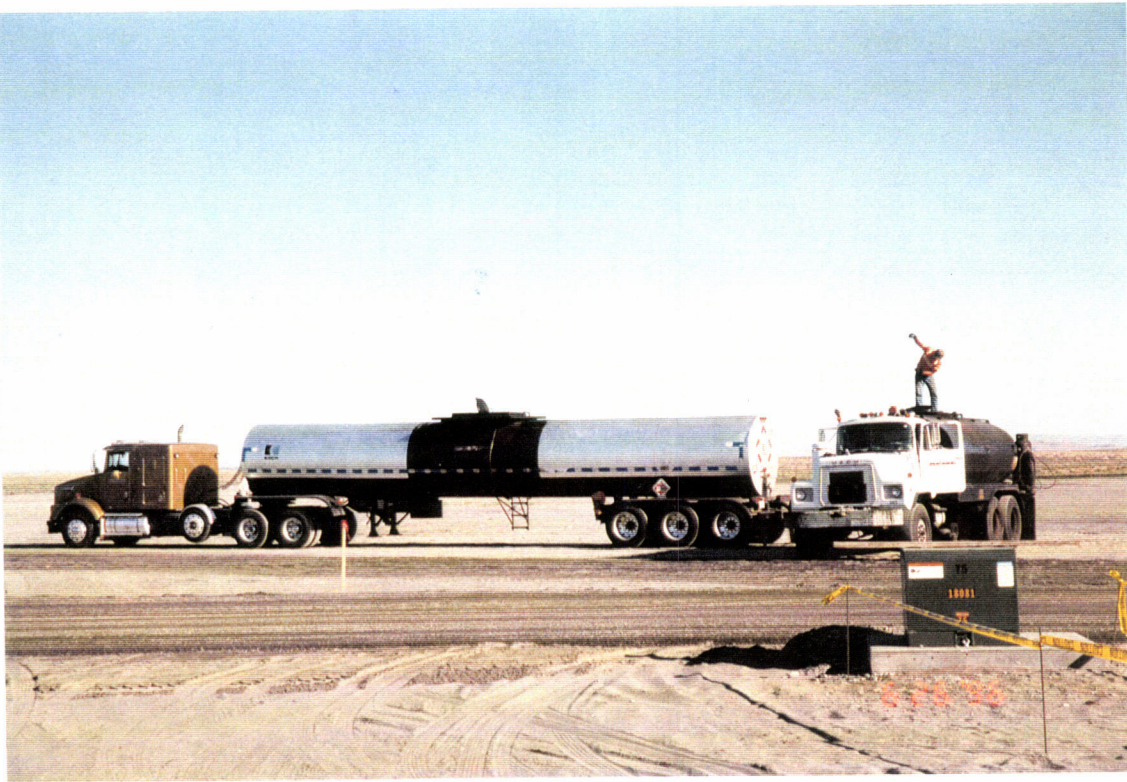
Loading MC-250, the first layer of the multiple layer bituminous road surfacing.
