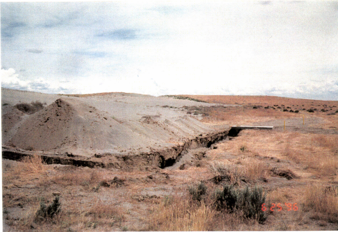
Duct bank trench for the chiller pad at the southwest arm End Station.
