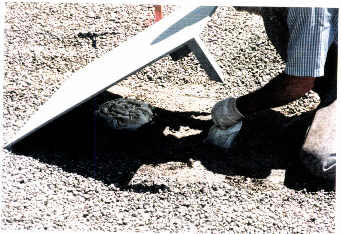
View of underside of the plate cover, conduits are sealed with a foam plug.
