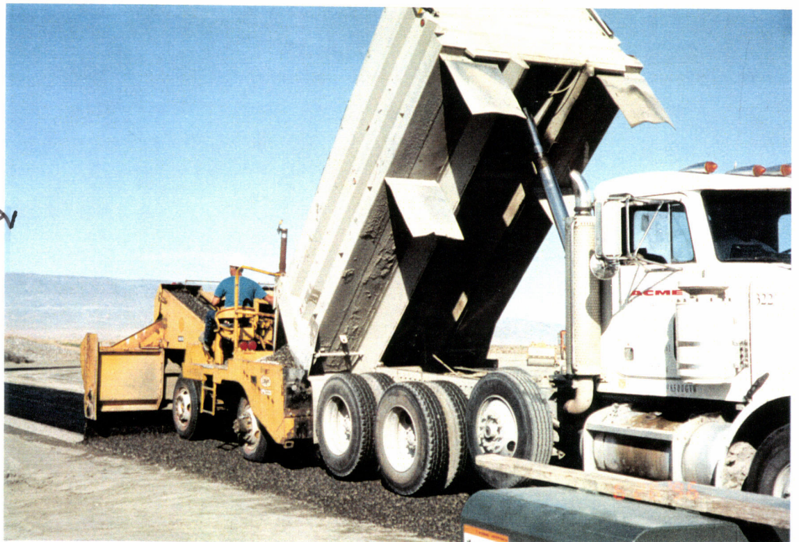
Another view of the gravel spreading equipment being loaded with gravel.
