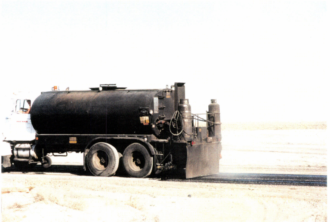
Spraying MC- 250 for the temporary access road around the Corner Station.
