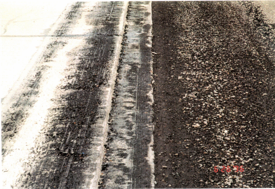
View of the alignment groove showing that cutting was limited to the areas where the alignment groove finished elevation was out of tolerance.
