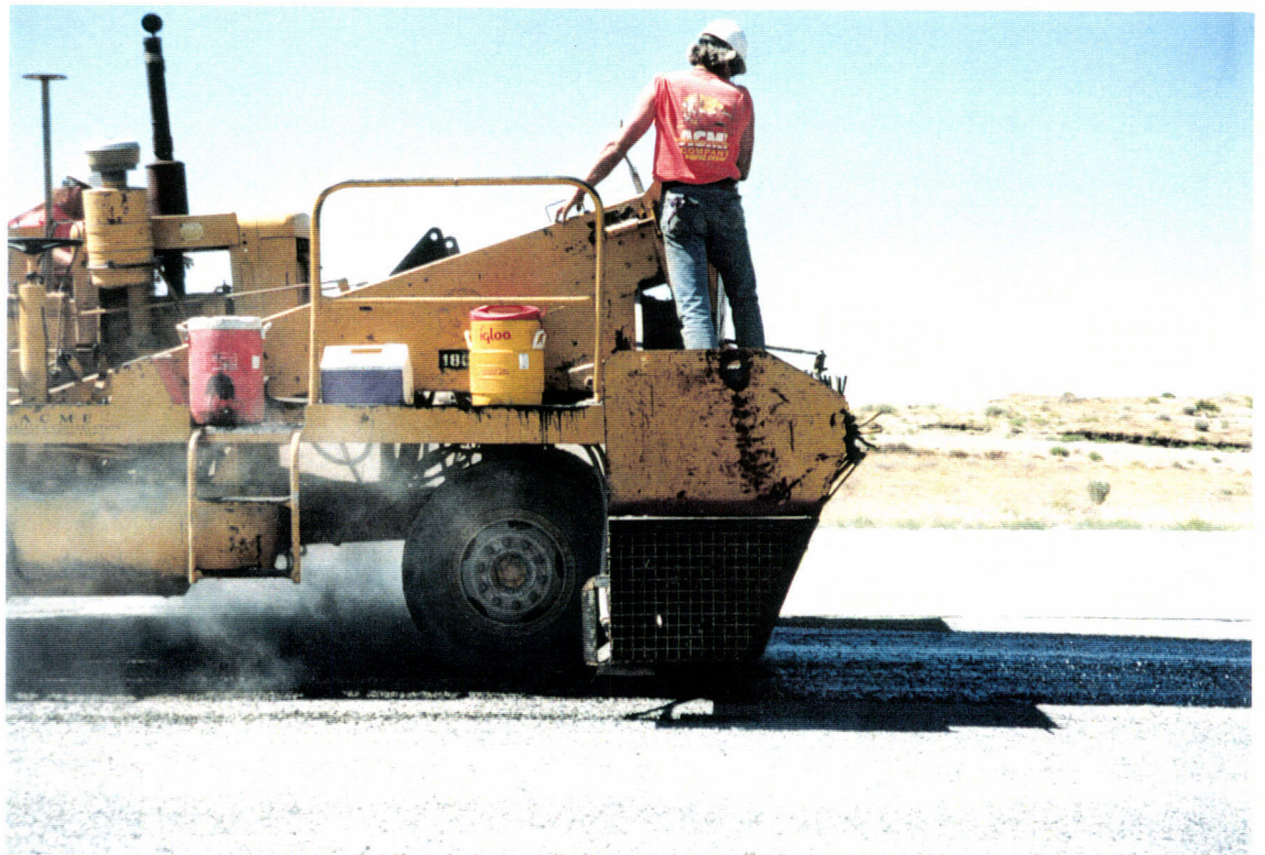
Following placing the second and final layer of gravel along the southwest arm.
