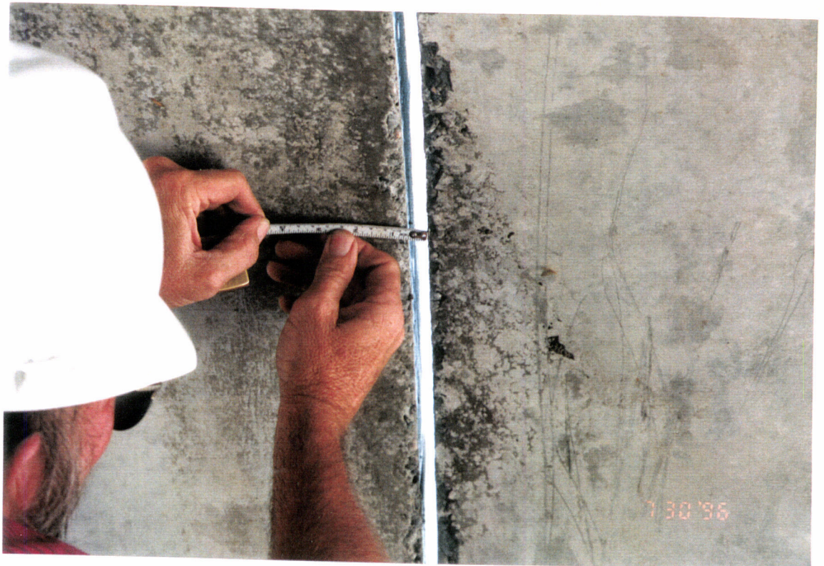
10- Verifying the fit up of Beam Tube Enclosure modules.
