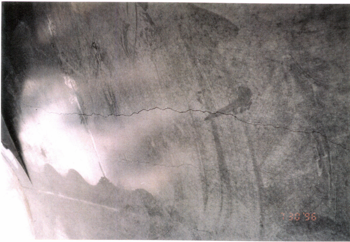
5- Close up of the crack in the Type 'A' enclosure.
