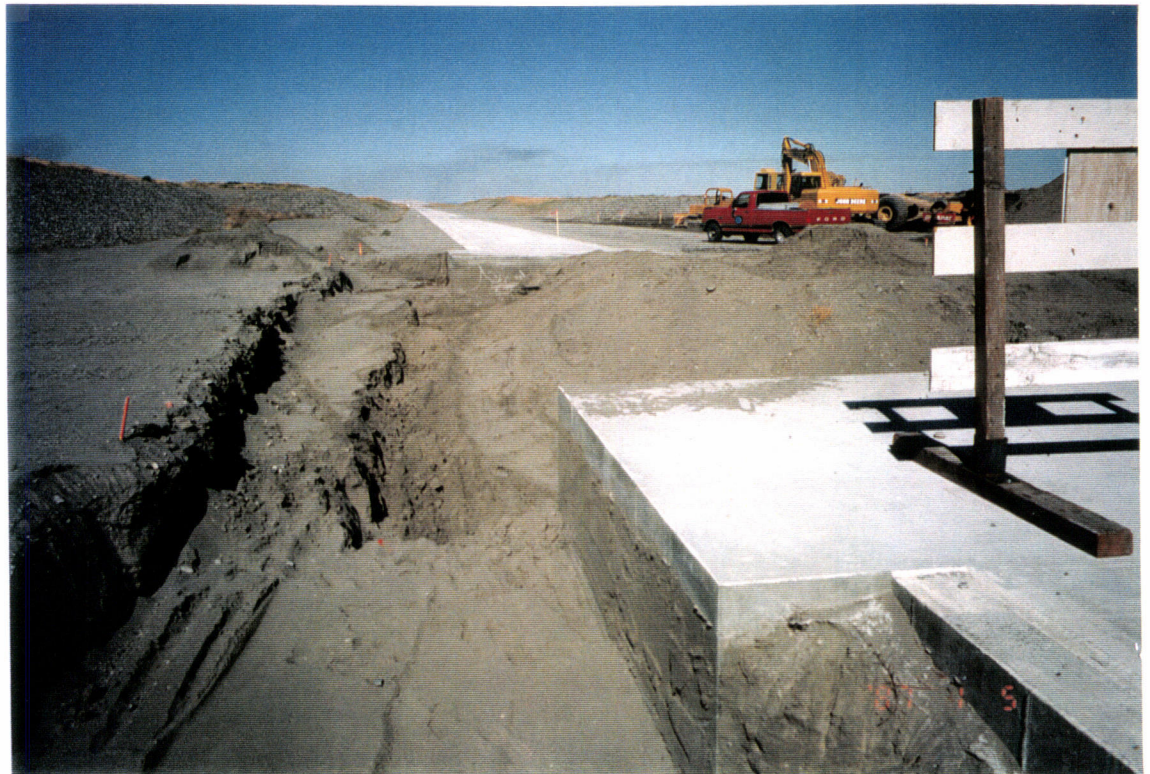
21- Excavation continues at the SW mid station.
