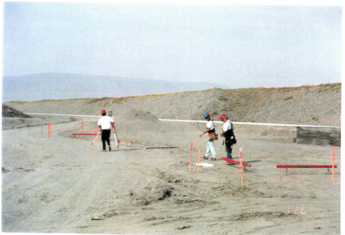
28- Marking area for the pads and footings at SW mid station.
