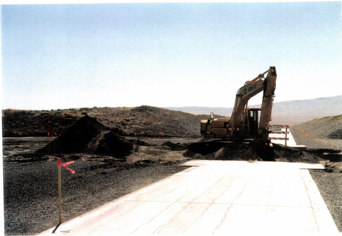
20- Excavation begins for the technical slab at the SW mid station.
