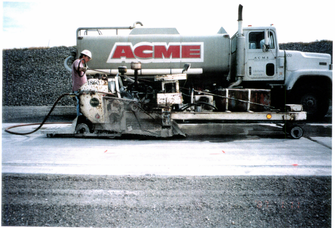
34- Grinding high points on the NW arm beam tube slab, in preparation for beam tube supports.
