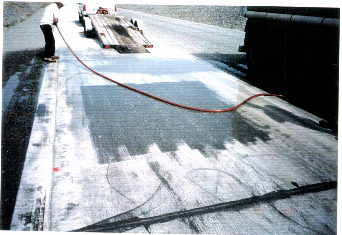
38- Completed grinding on the beam tube slab.
