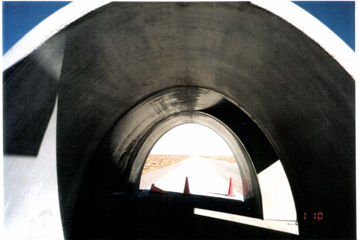
12- A view looking through the three enclosures while in place on the beam tube slab.
