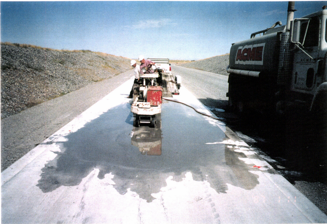
37- Grinding of the beam tube slab in progress.
