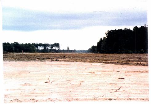
22. Northwest quadrant at center section showing the results of back dragging to remove puddles.
