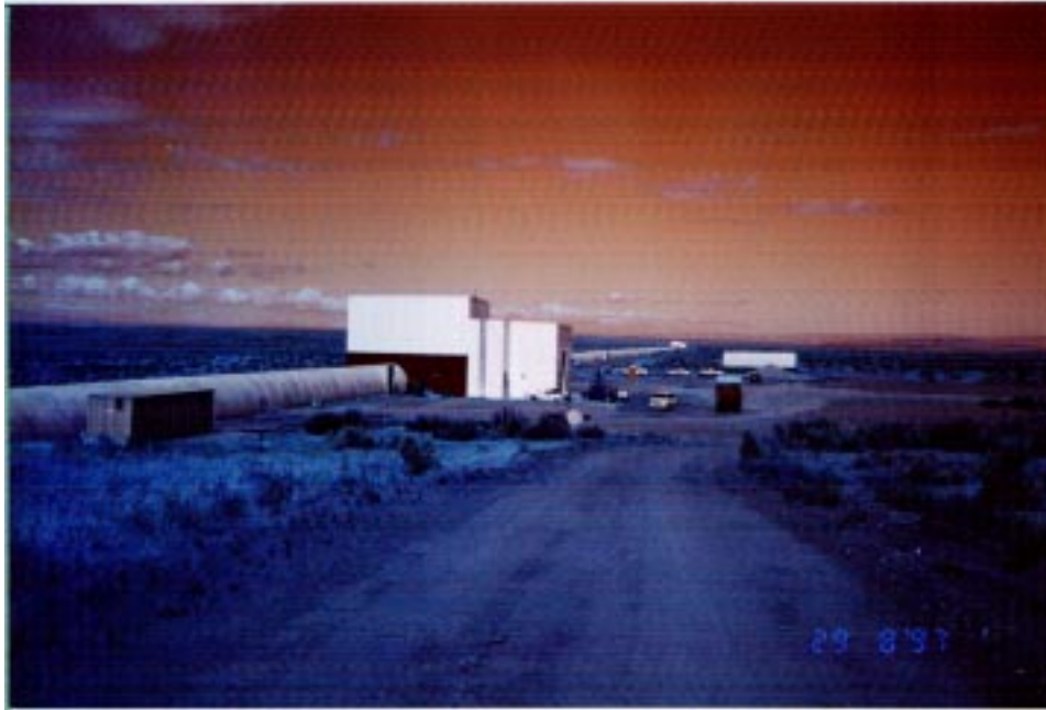
Figure 10. View of the Completed Beam Tube Enclosure on the 'X' (Northwest) arm at the Hanford Site.
