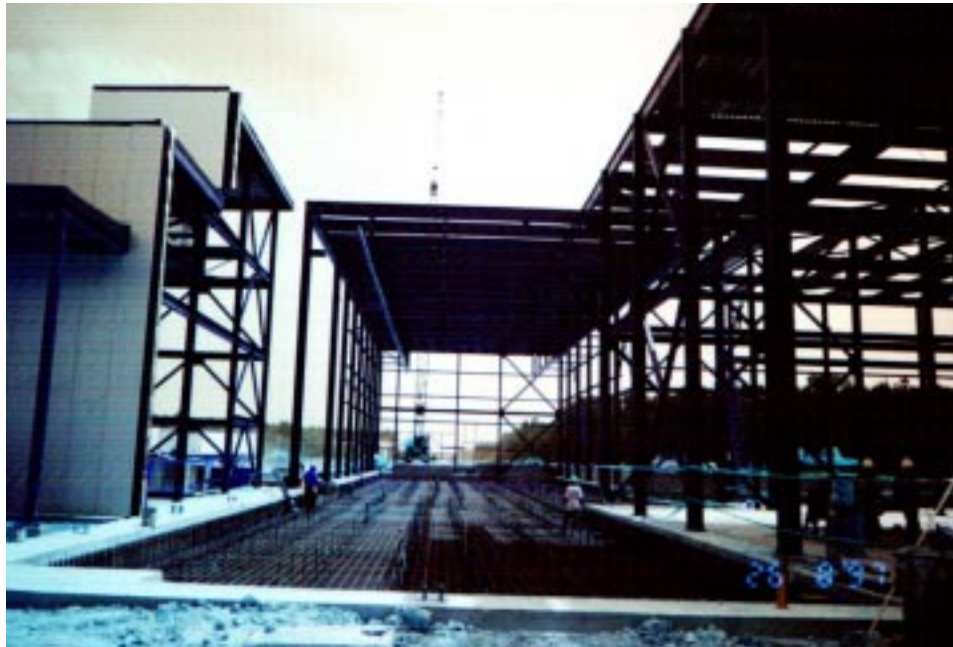
Figure 16. View of Steel Framing of the Corner-Station at the Livingston Site.
