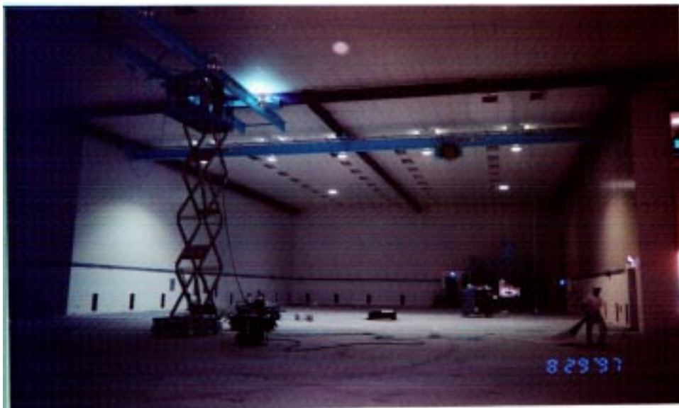
Figure 15. View of Inside of LVEA at the Corner-Station at the Hanford site.
