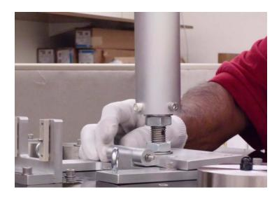
2.2.9 Attach four 1/4-20 SHCS through **Top Hinge Plate** on **Suspension Assembly** to **Bottom Hinge Plate** on **Baffle Box Assembly**.
