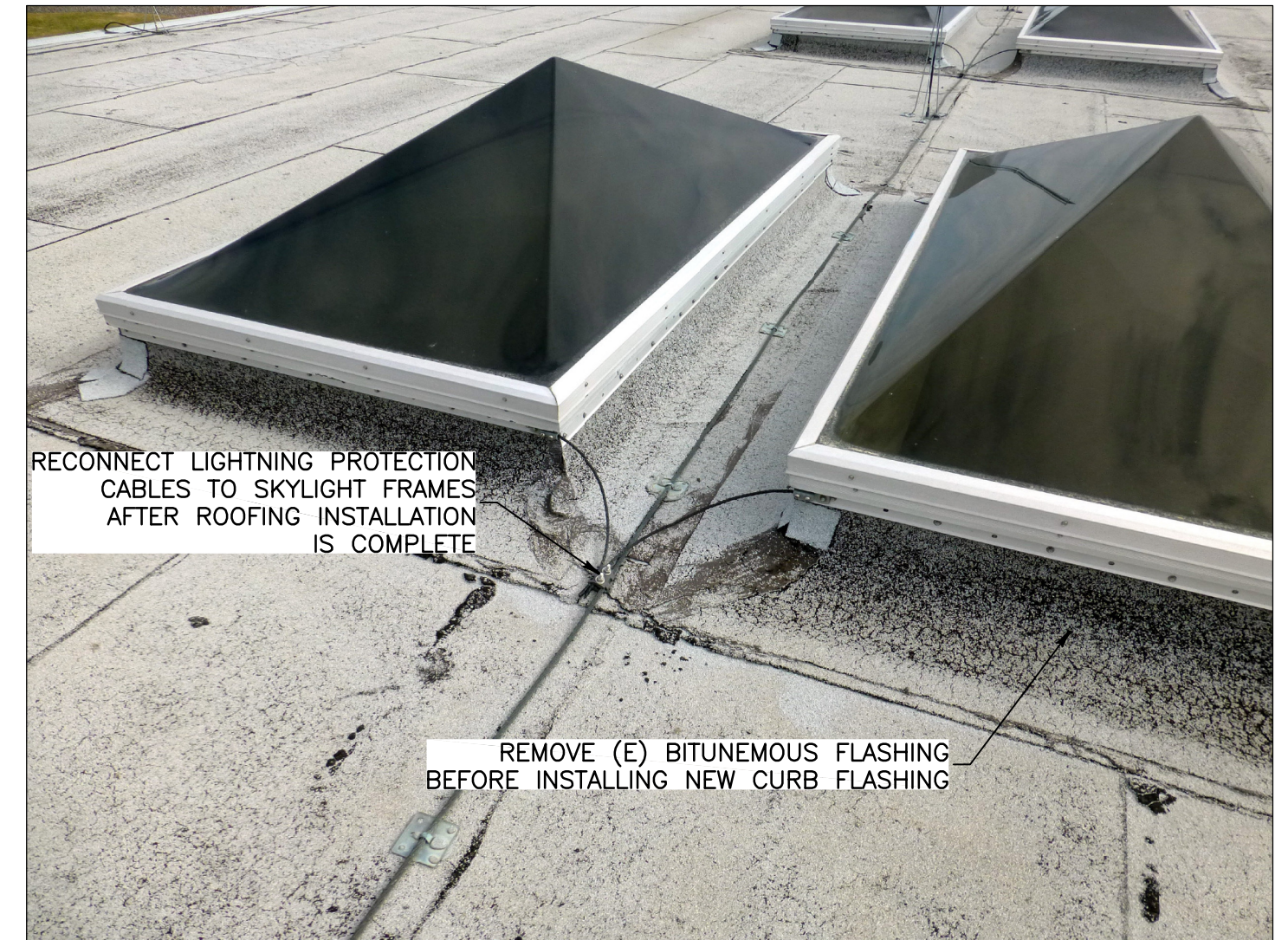
PHOTO 6 SKYLIGHT PERIMETER CONDITION REF
