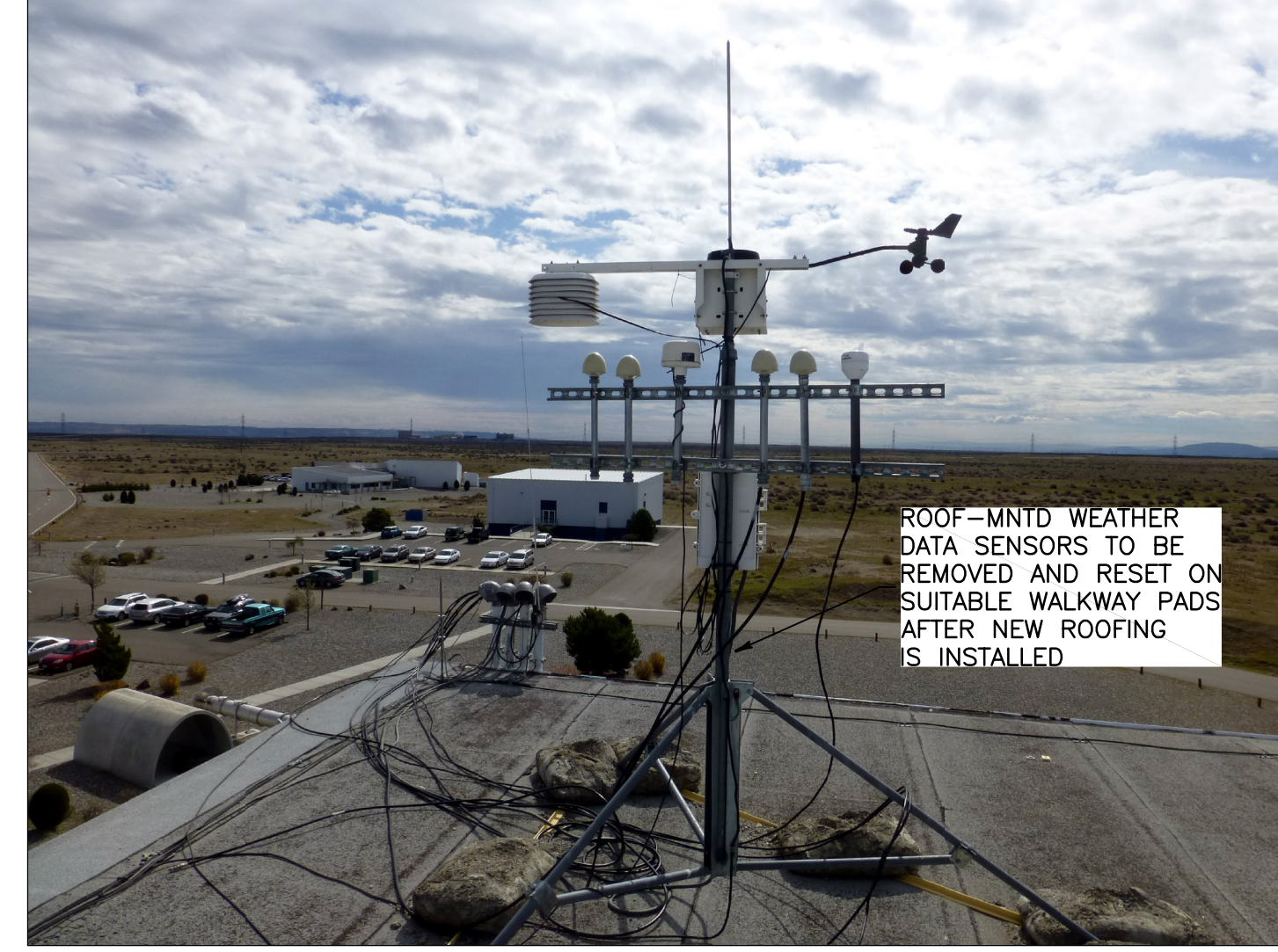
PHOTO 9 METEOROLOGY STATION CONDITION REF
