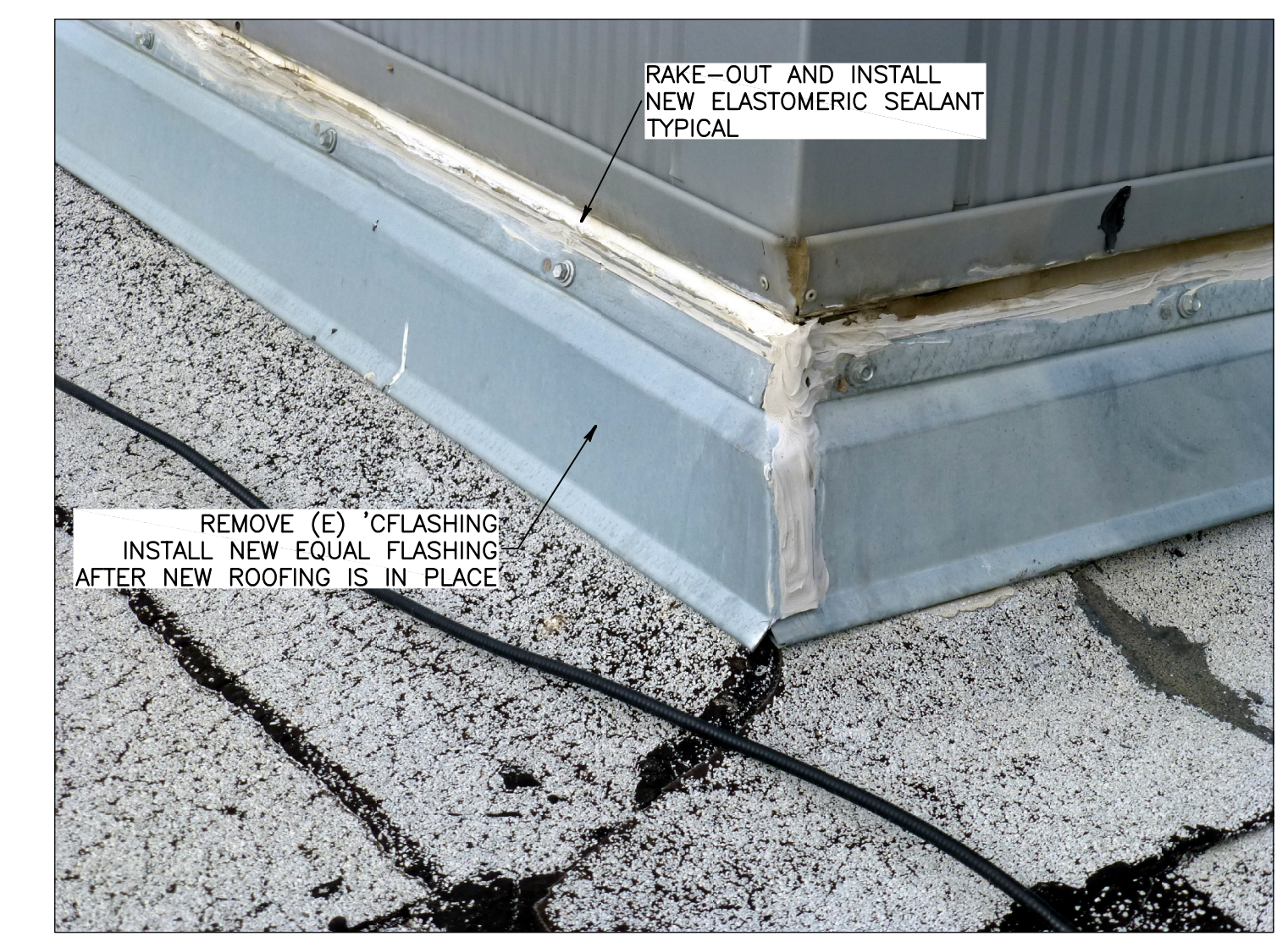
PHOTO 4 FLASHING DETAIL REF
