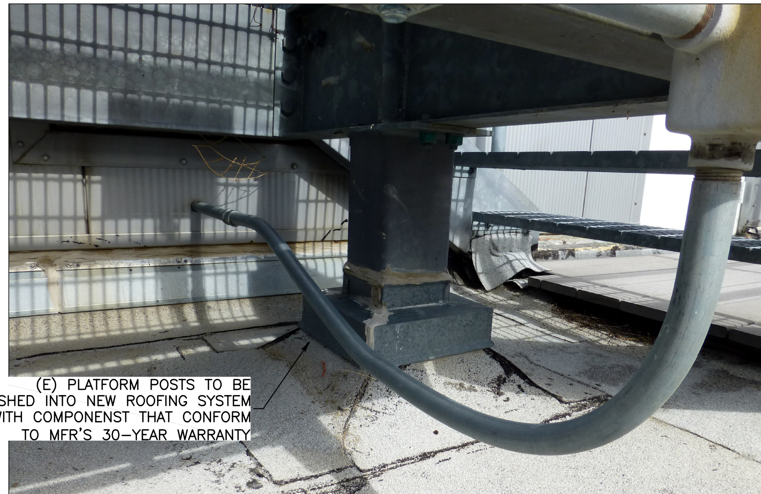
PHOTO 12 EXISTING PLATFORM PEDESTAL CONDITION
