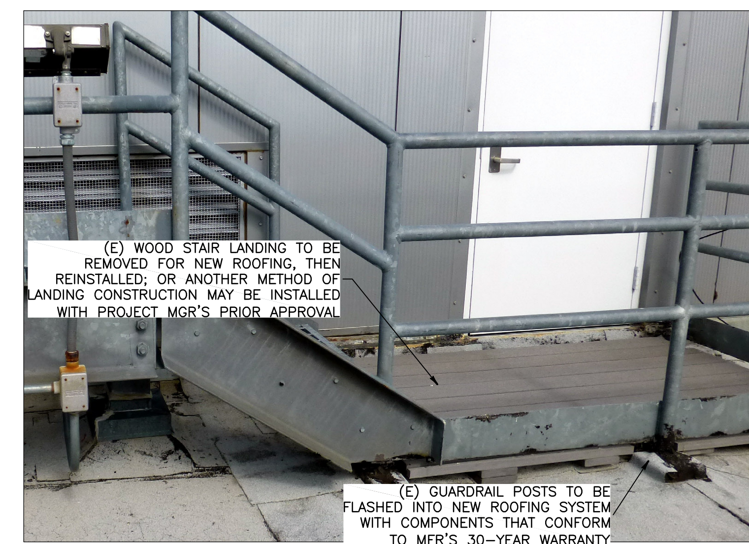
PHOTO 13 EXISTING LANDING CONDITION REF
