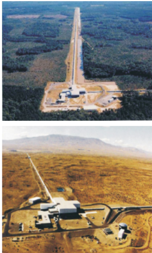
FIG. 4. Images showing the two LIGO sites in Livingston, Louisiana (top) and Hanford, Washington (bottom). The interferometer arms in each detector are 4 km long and contain vacuum pipes along the whole optical path [6].
