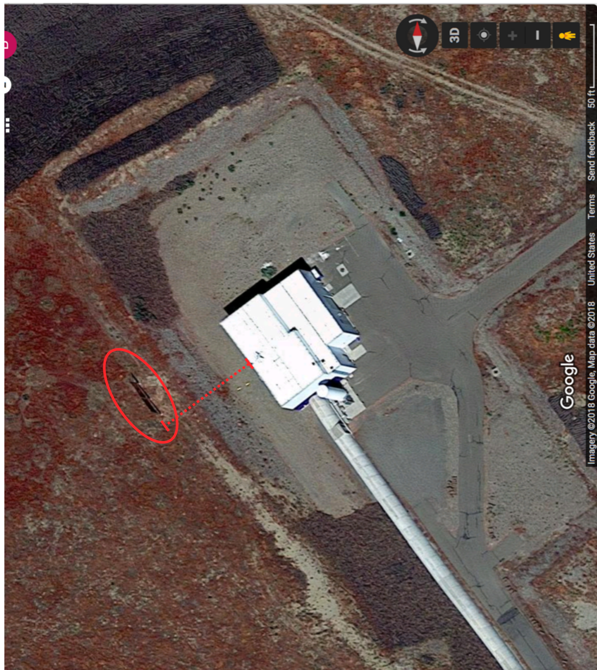
Google image of LHO EndX, Test fence is visible, Test fence is ~85 ft from the building. Top of the test fence is about 5 feet below the top of the building.
