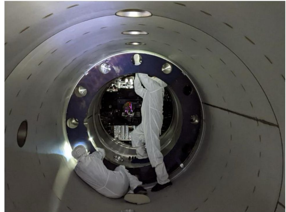
Installing baffles to hide small flanges
