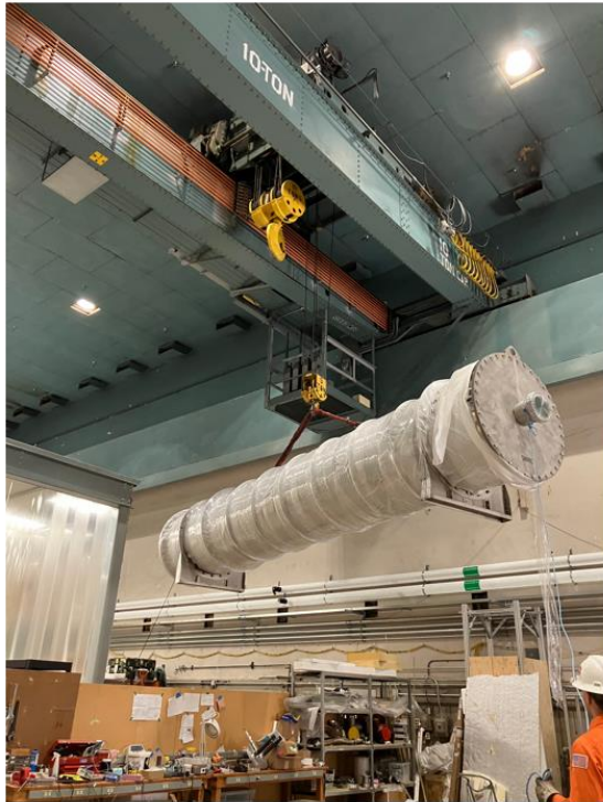
Craning chamber into place at Caltech synchrotron building
